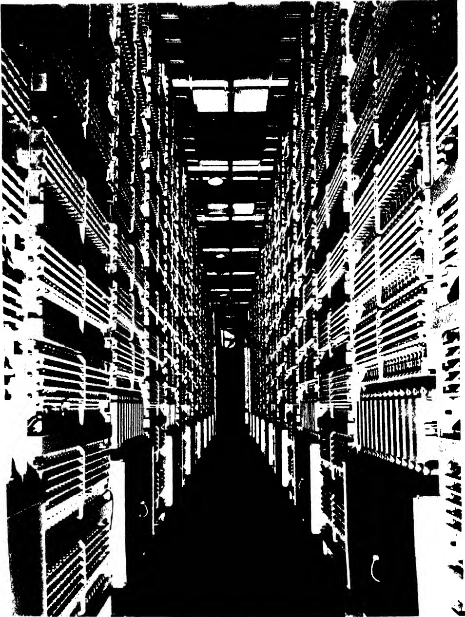
FIG. 14. AN AISLE OF A CENTRAL OFFICE IN A DIAL SWITCHING AREA SHOWING COMPLEXITY OF MODERN TELEPHONY.
